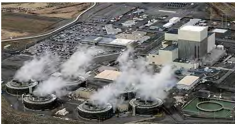
Figure 20. Columbia Generating Station (Previously called WNP-2 Nuclear Power Plant)
