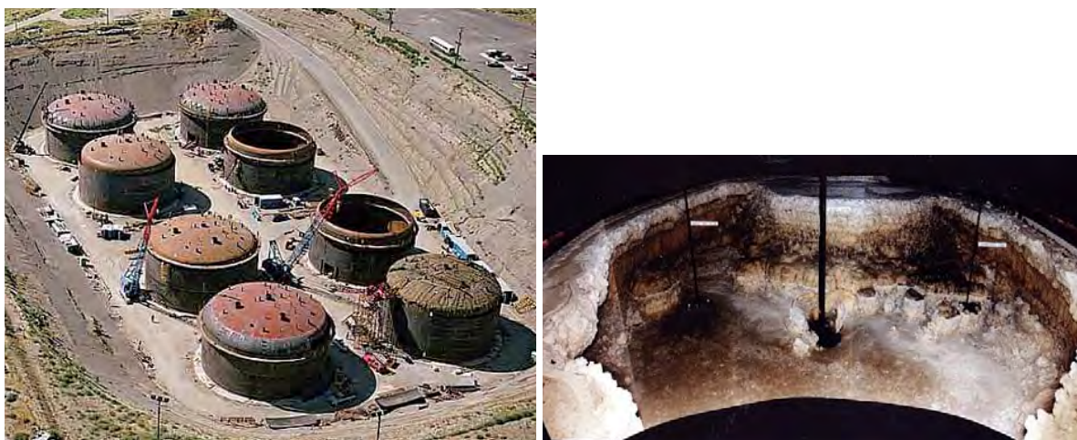
Figure 4. 177 underground storage tanks (right figure) and crust of radioactive tank waste (left figure)
